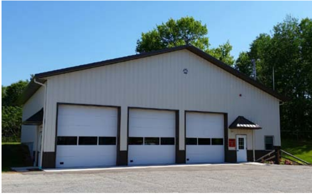
Annex at Station 1, Admin offices
