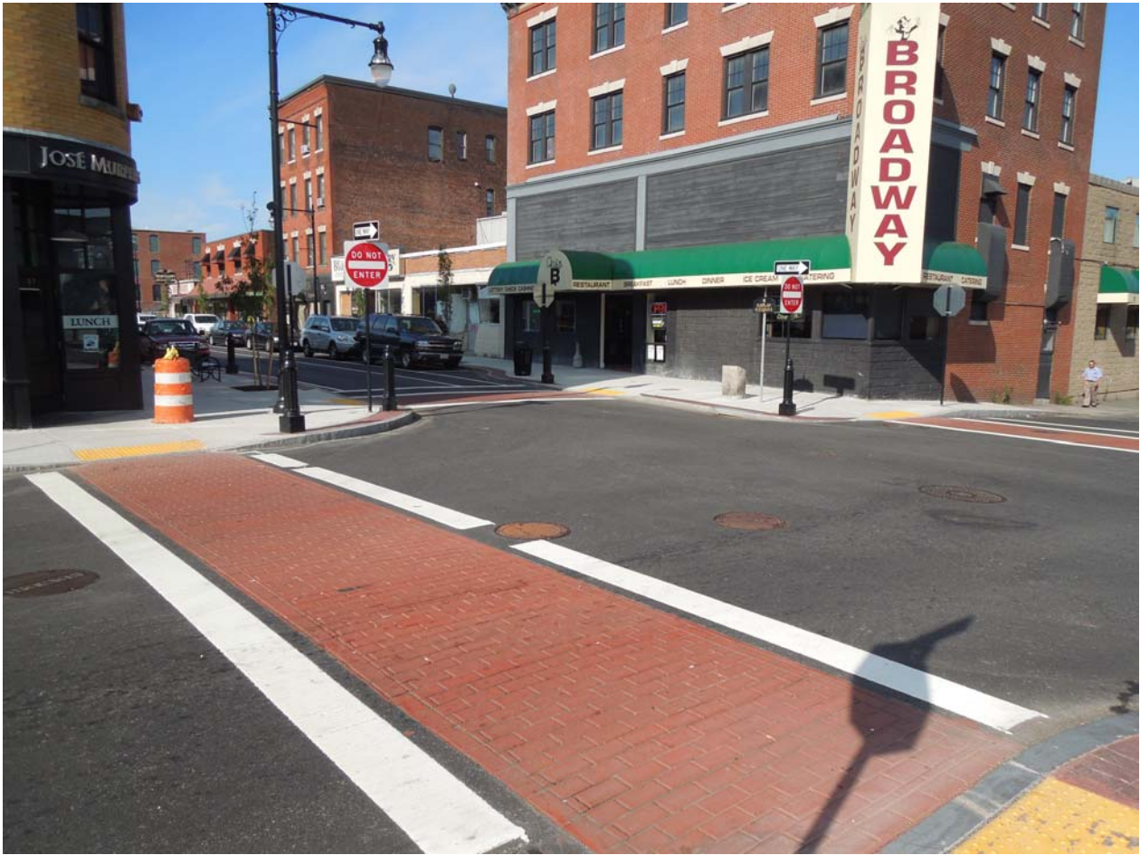
2012 Worcester Canal District Post-Construction Photos 018
