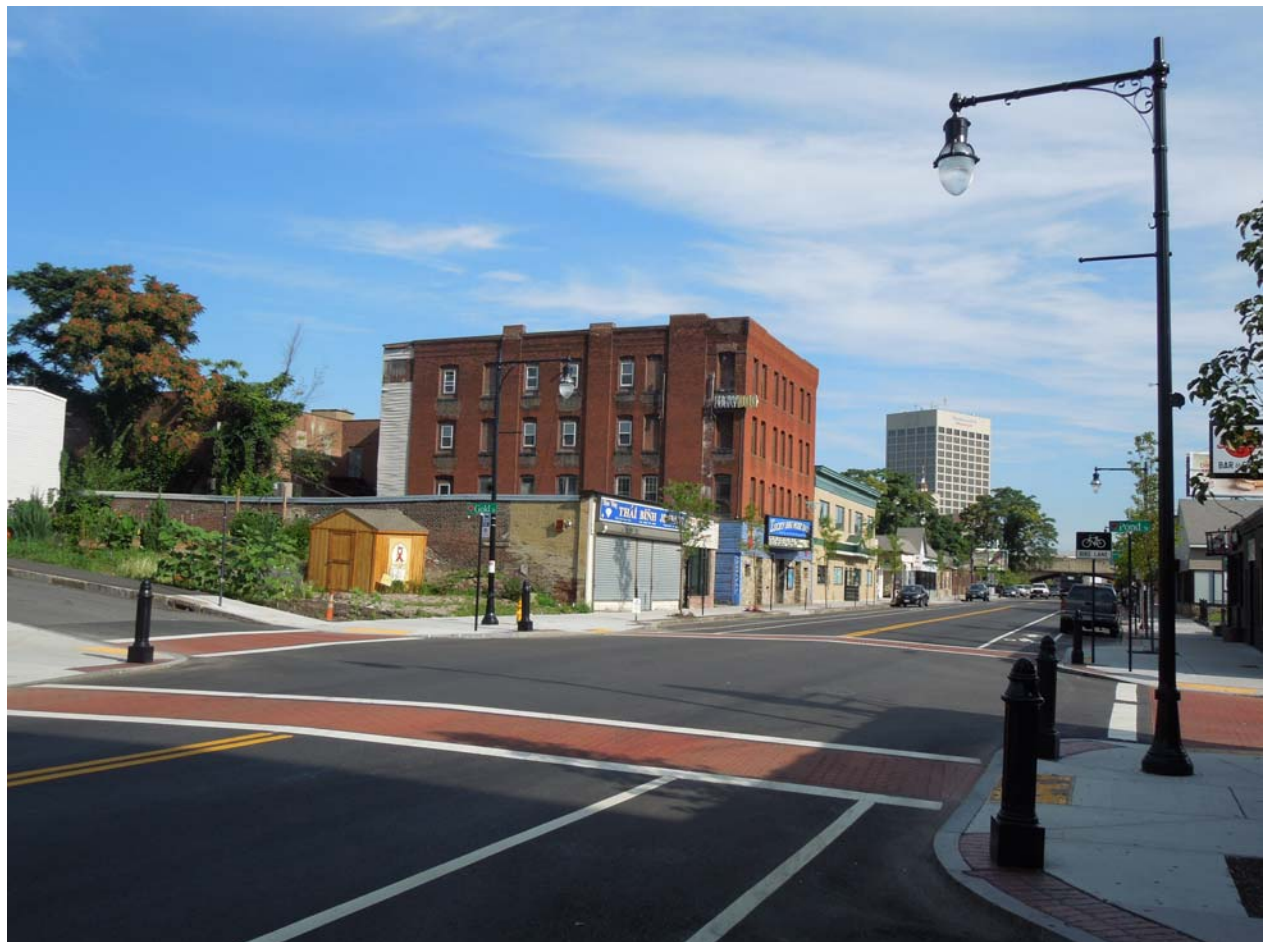
2012 Worcester Canal District Post-Construction Photos 012
