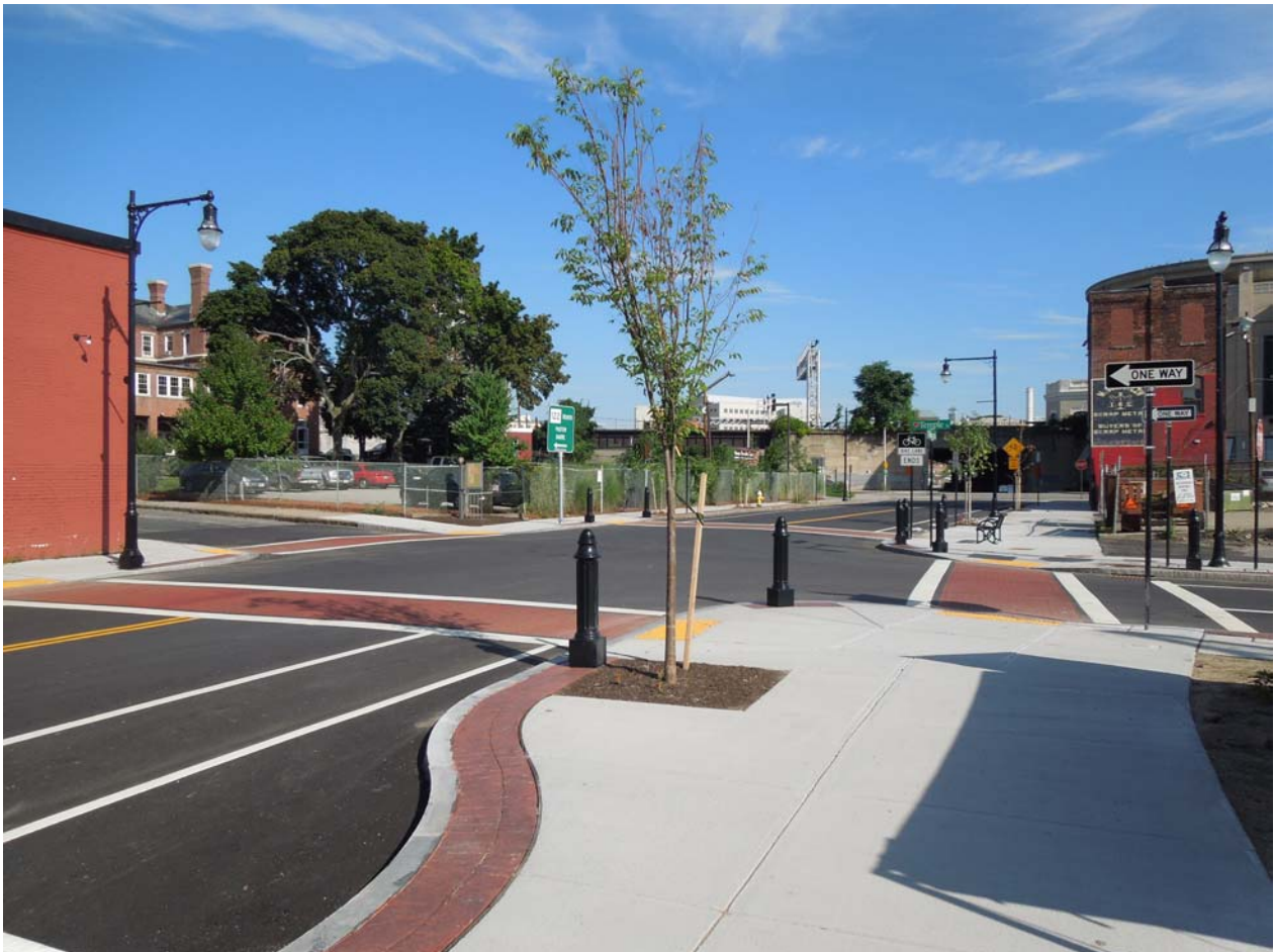
2012 Worcester Canal District Post-Construction Photos 024
