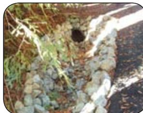
**D** A rocked or vegetated swale lining the edge of a road or driveway reduces erosion potential by SLOWING runoff and then SINKING it back into the soil or directing it to a safer outlet (page 29).
