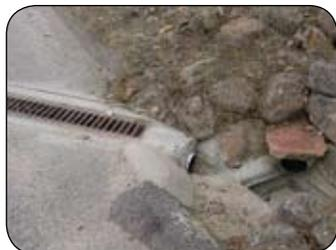
**MAINTENANCE:** Ensure that the grate is open before and during storm events (not covered by leaf litter). Check that the outlet is protected, non-eroding, and clear of debris and sediment so water drains freely.
