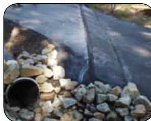
**B** An asphalt berm (like a small speed bump) known as a waterbar can be added to existing driveways to SLOW and SPREAD runoff to vegetated or rocked infiltration areas (page 35).
