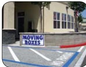
**C** Pervious concrete (pictured) or other materials such as paver stones or turf block, allow water to SINK into the soil decreasing runoff (page 31).
