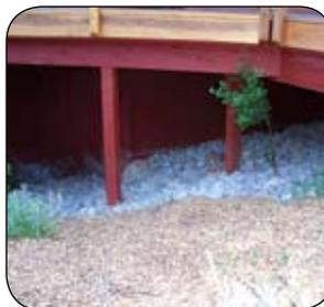
**B** Adding drain rock **SLOWS** runoff and safeguards the drip-line area under elevated surfaces. Mulch around the perimeter adds extra protection to the surrounding bare soil (pages 22-23).
