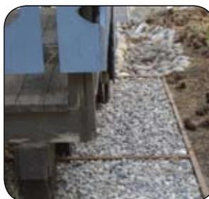
**A** Adding drain rock or vegetation to the perimeter **SLOWS** and **SPREADS** water limiting the transport of sediment (pages 22-23)
