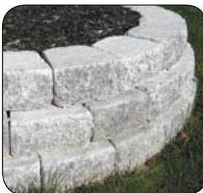
**C** Terracing or retaining walls may be added to sloped areas to keep rock or other mulch in place and protect hillsides (pages 36-37)
