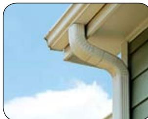
**A** Adding gutters and downspouts works to direct water to a safe location away from bare soil and buildings (see page 20).
