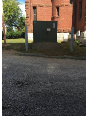
Pad Mounted Transformer at Library
