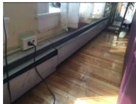
Typical Fin Tube Radiation
