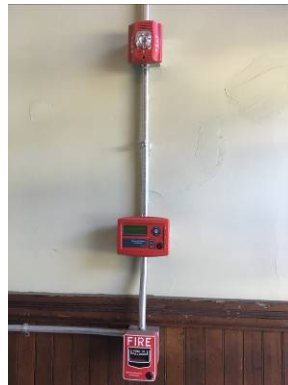
Remote LCD Annunciator
