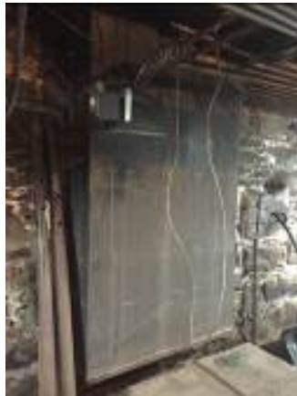
Combustion Air Duct
