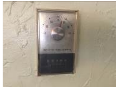
Typical Standalone Thermostat
