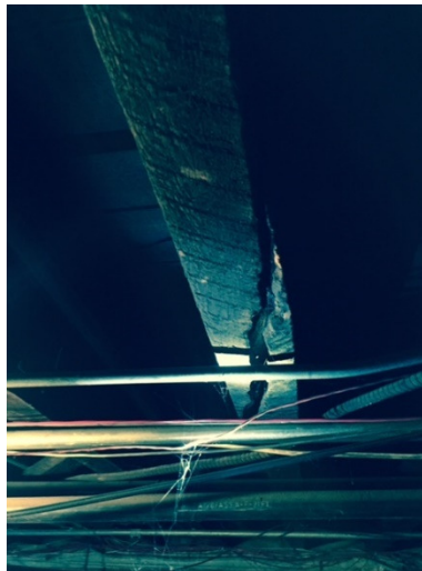
Splitting, cracking and improperly supported joists (first floor framing)
