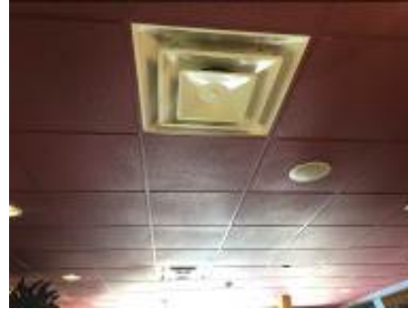
Typical Supply Air Diffuser
