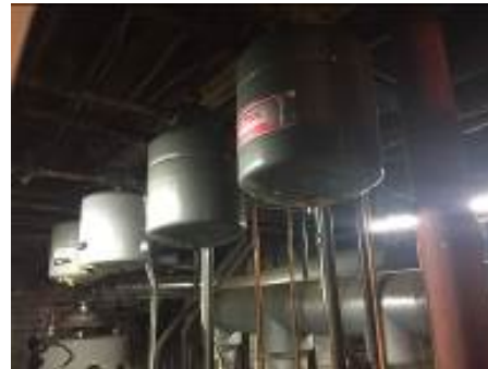
HW Expansion Tanks
