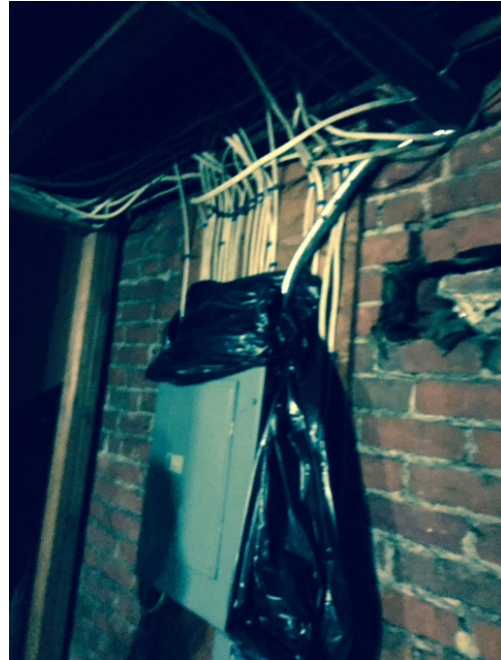
Leak issues at basement electric panel
