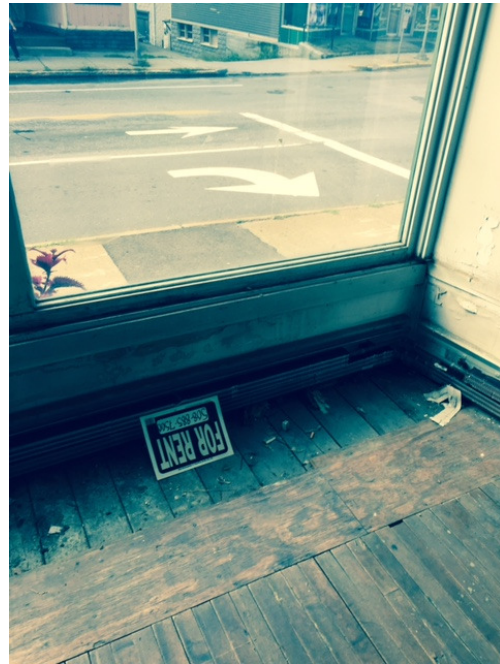
First floor – deteriorated floors
