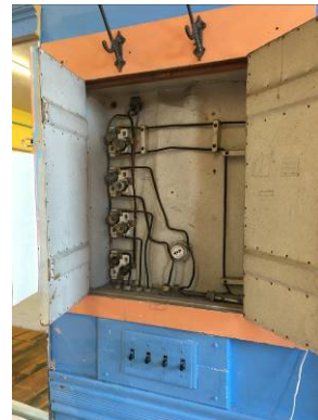
Flush Fusible Knob & Tube Panel
