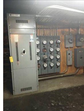
Main Breaker & Meter Center
