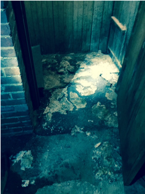
Repeat sewerage issues at basement
