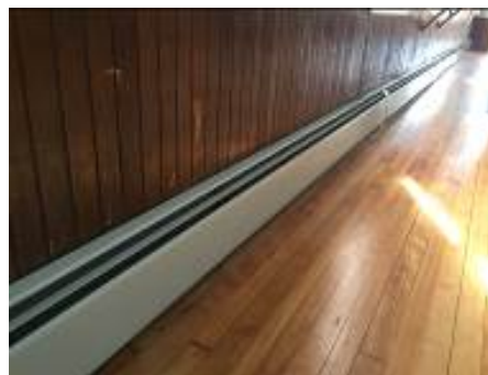
Typical Fin Tube Radiation
