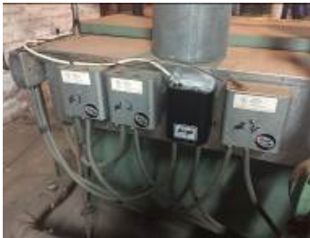
Boiler Control Relays
