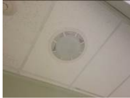
Typical Ceiling Exhaust Fan
