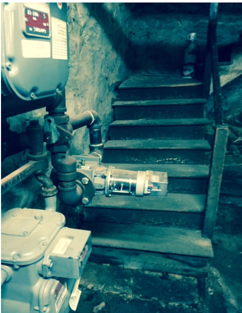
Gas meter blocking stair run at basement
