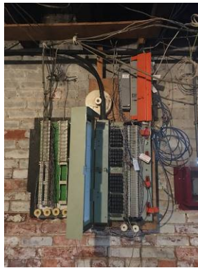
Telephone Demarcation in Basement
