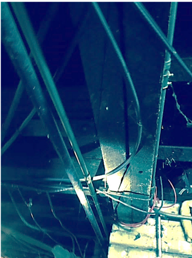
Splitting, cracking and improperly supported joists (first floor framing)
