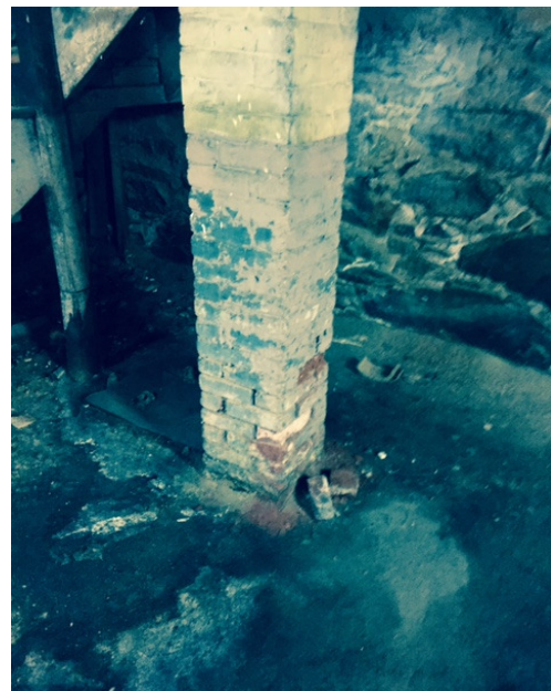
Deteriorating brick pier in basement
