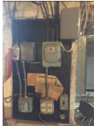
Time Clock & Combustion Air Damper Switch
