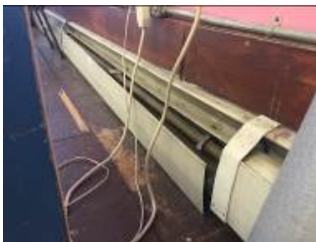
Typical Fin Tube Radiation
