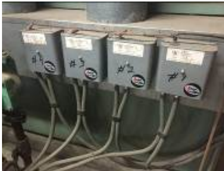
Boiler Control Relays
