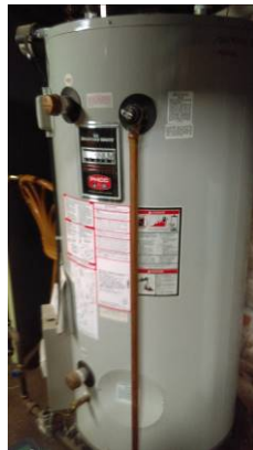
Gas-Fired Water Heater
