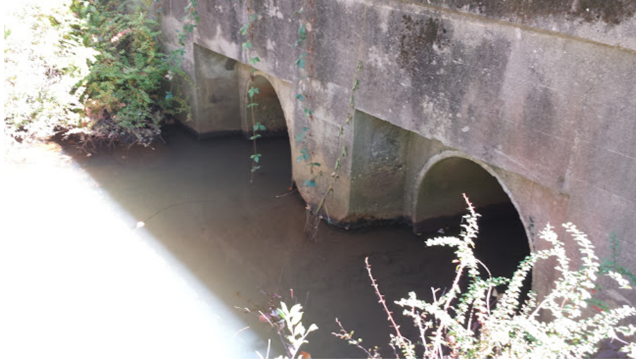
Figure 6: Double-Pipe Culvert (Photo: Ryan Bagge, 2014)
