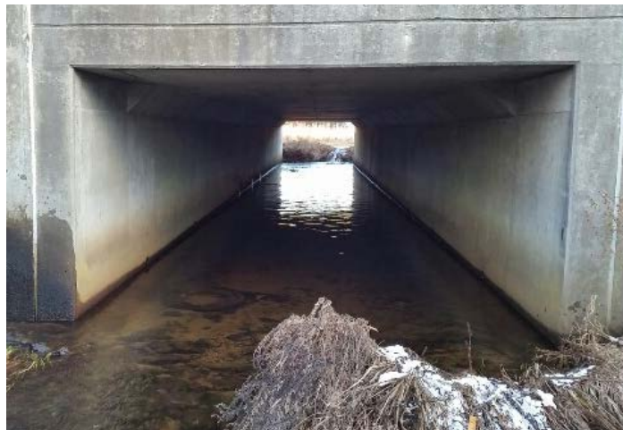
Figure 9: Pre-cast Box Culvert (Photo: Ryan Bagge, 2014)
