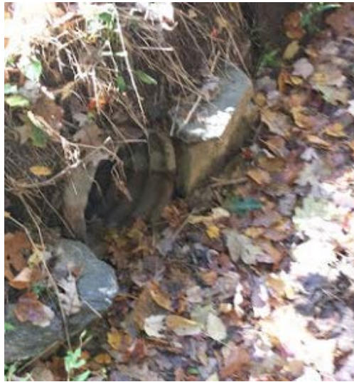
Figure 2 - Corrugated Metal Pipe Culvert (Photo: Ryan Bagge, 2014)
