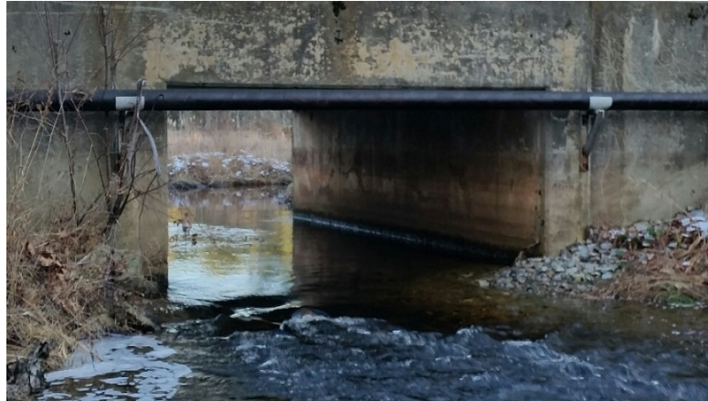
Figure 8: Open-Bottom Box Culvert (Photo: Ryan Bagge, 2014)
