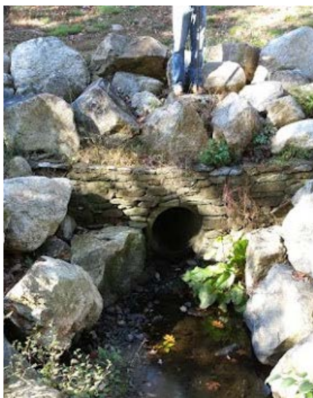
Figure 5: Concrete Pipe Culvert (Photo: Ryan Bagge, 2014)
