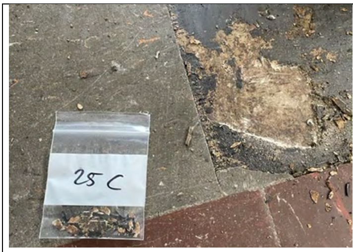
26. View of 12x12 black floor tile
