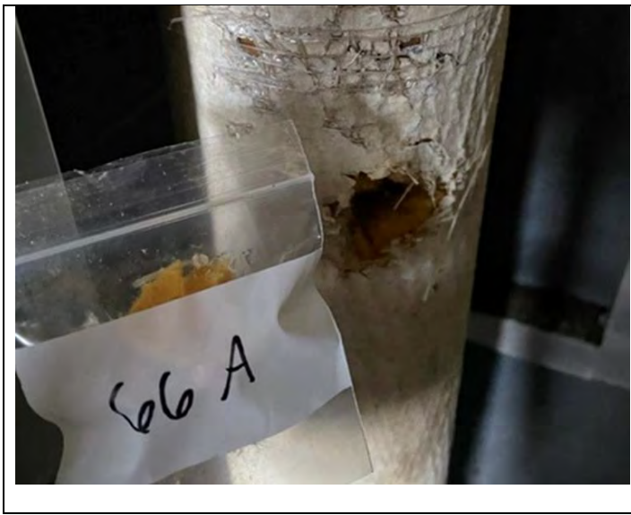
67. View of new fiberglass TSI
