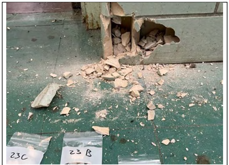
24. View of green wall tiling and grout
