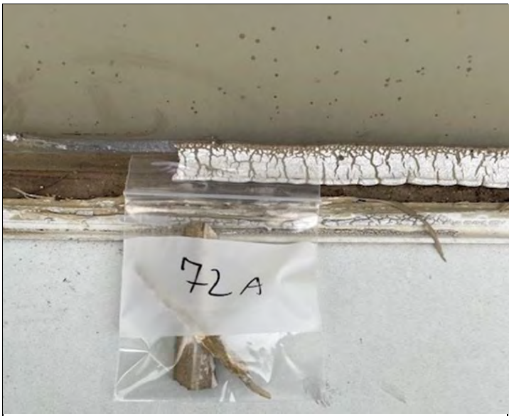
73. View of exterior white caulking old
