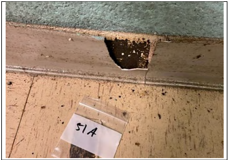
52. View of 4" tan base board 1977
