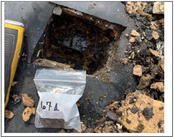
68. View of roof coring (TPO on top of EDPM)
