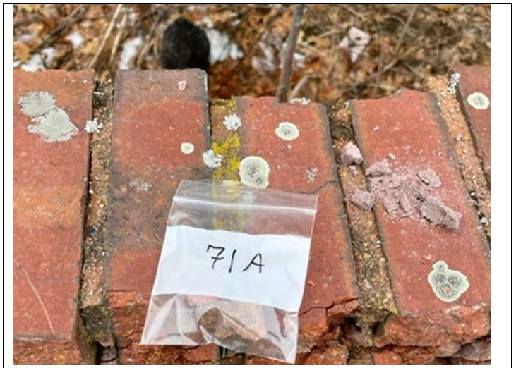
72. View of exterior brick and mortar
