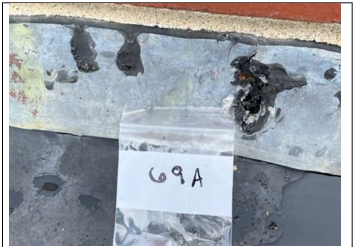
70. View of black chimney caulking
