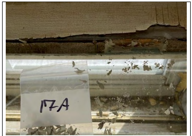
18. View of window caulking
