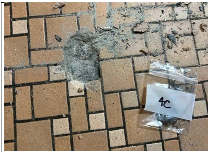
5. View of bathroom floor tiling, mortar, and grout
