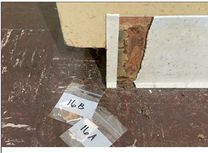
17. View of 6" white base board
