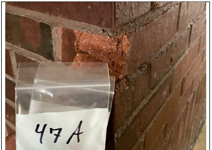
48. View of 1977 brick and mortar
