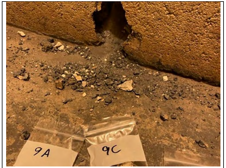
10. View of cinder block.
