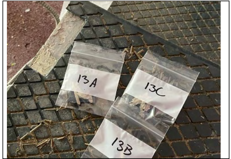
14. View of blue stair treads
