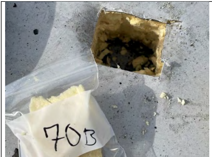
71. View of white new roof coring
