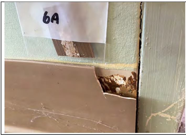
7. View of 6" tan base board
