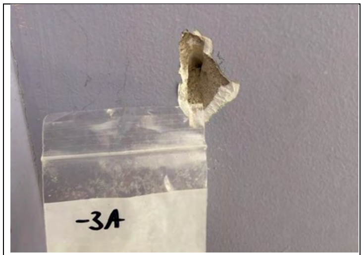
4. View of dry wall
