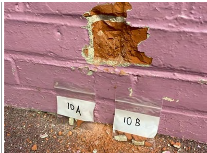
11. View of brick and mortar
