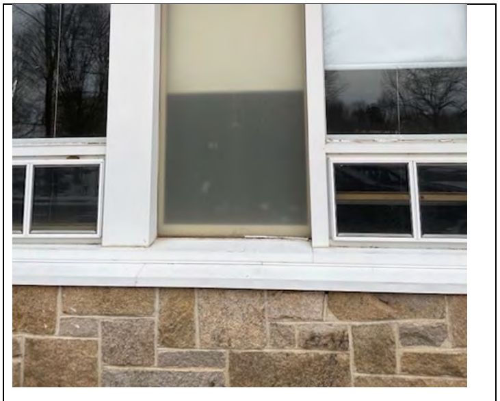
74. View of white exterior window caulking new
