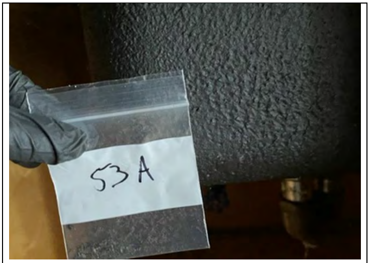
54. View of black under sink coat
