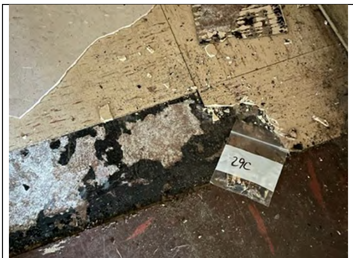
30. View of 12x12 yellow flooring tile
