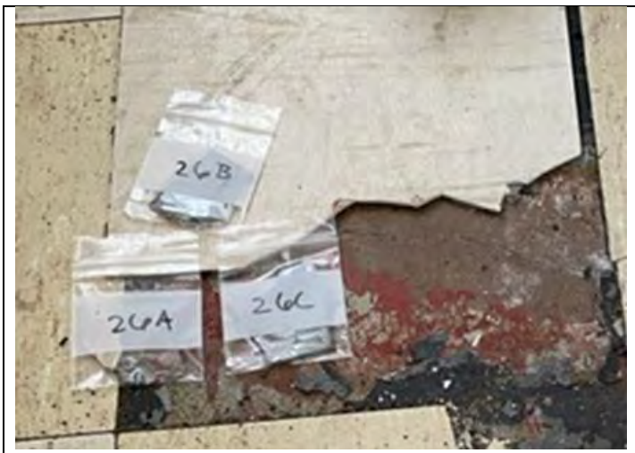
27. View of 12x12 white floor tile
