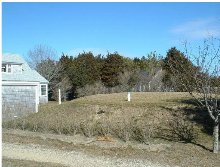
FIGURE 2-2 MOUNDED SEPTIC SYSTEM
