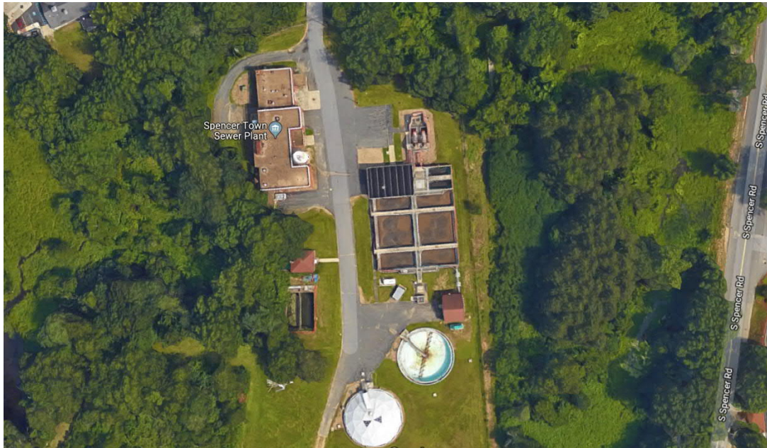
FIGURE 3-2 SPENCER WASTEWATER TREATMENT PLANT
