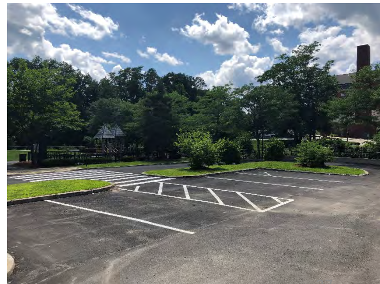
Repave parking spaces and directional arrows
